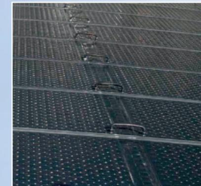
APSOfluid® ASSIWELL® metal hoses connect solar thermal collectors.
